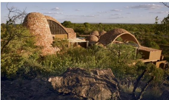
Figure 7: Mapungubwe Interpretation Centre, Zimbabwe, by Peter Rich Architects
