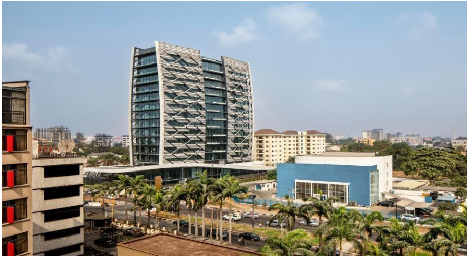
Figure 2. Kingsway Tower, Lagos – Nigeria.
