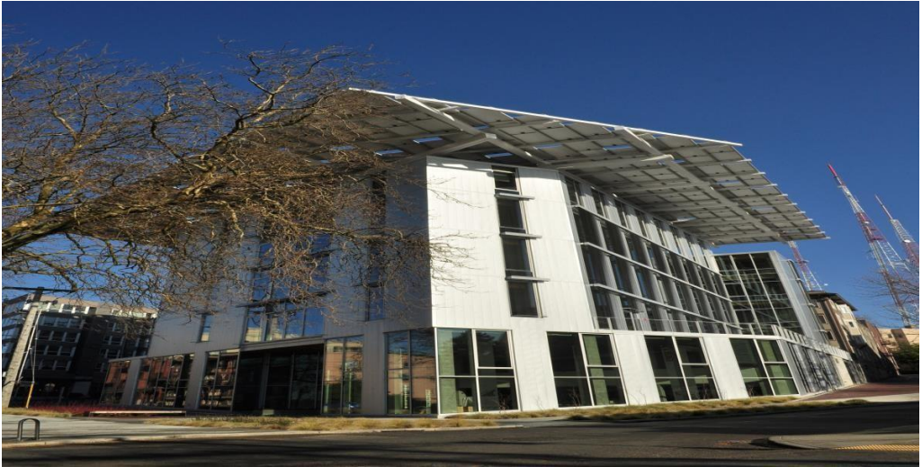
Figure 7. Bullitt Centre, Seattle-Washington in USA.
