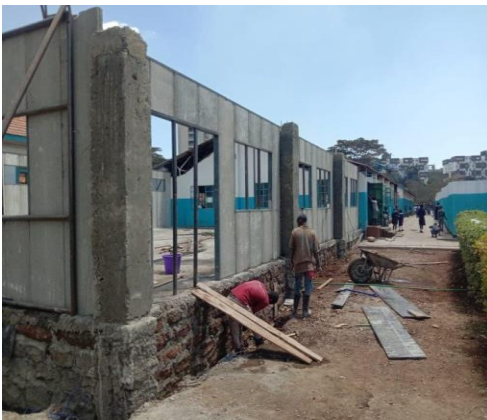
Figure 11: Precast Concrete Wall wall
