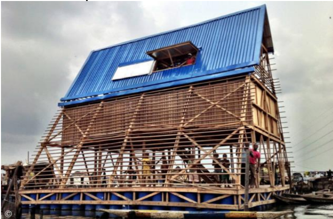
Figure 17: Makoko Floating School by NIé Architects
