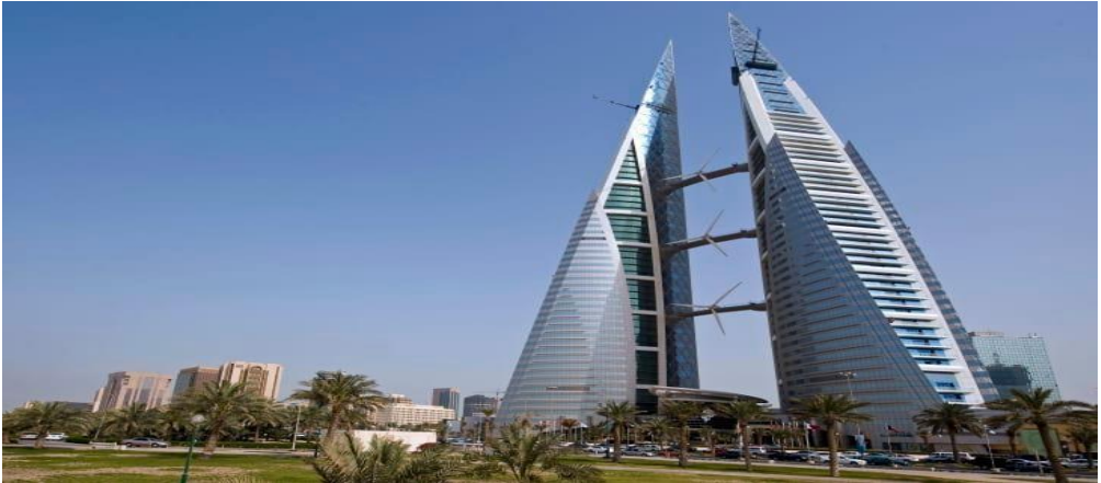
Figure 5. The Bahrain twin towers of the World Trade Center in Manama. Source: https://edition.cnn.com/style/article/green-buildings-world-sustainable- design/index.html
